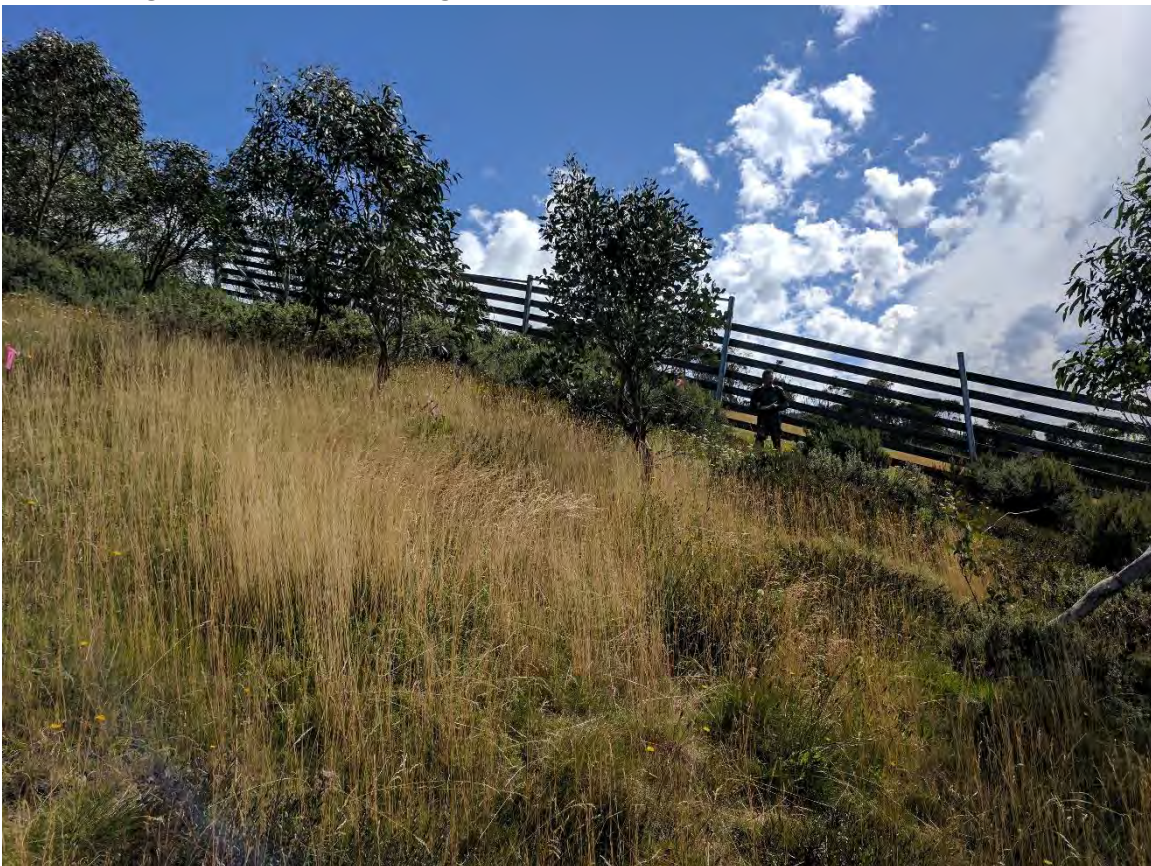
Figure 4: Section 2 - Corners to be re-aligned into the existing planted tree island on the side of the ski run
