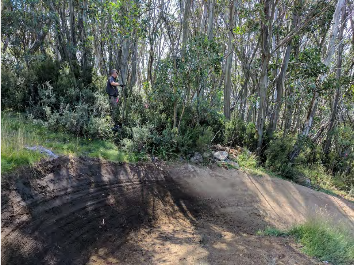
Figure 7: Section 4 – Relocate the corner into the vegetation on the side of the ski run
