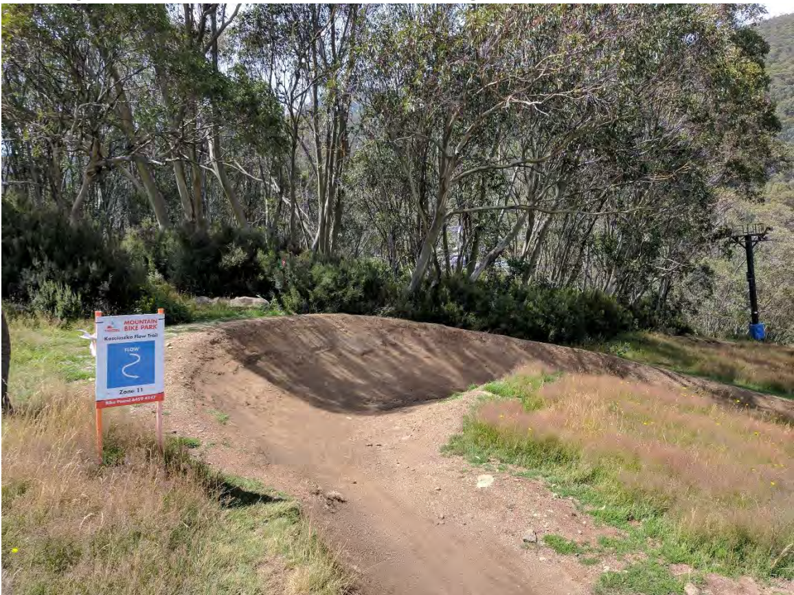
Figure 10: Section 6 - Relocate the corner into the vegetation on the side of the ski run
