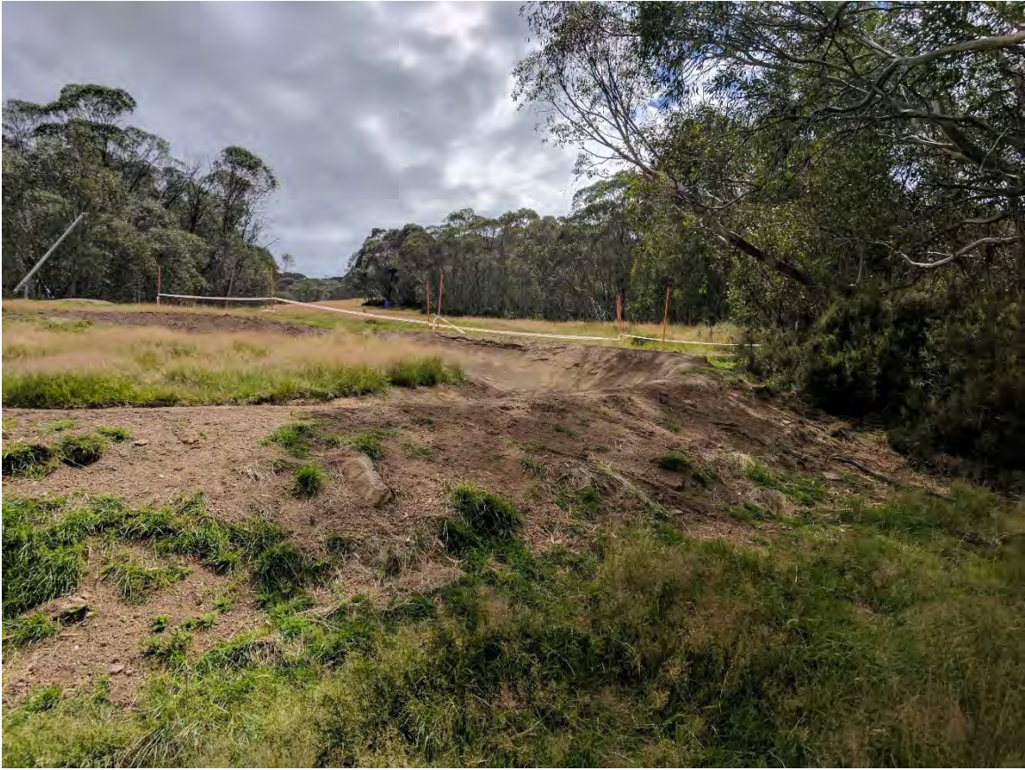
Figure 13: Section 8 - Relocate corner and berm off the ski slope into the vegetation on the side of the ski run
