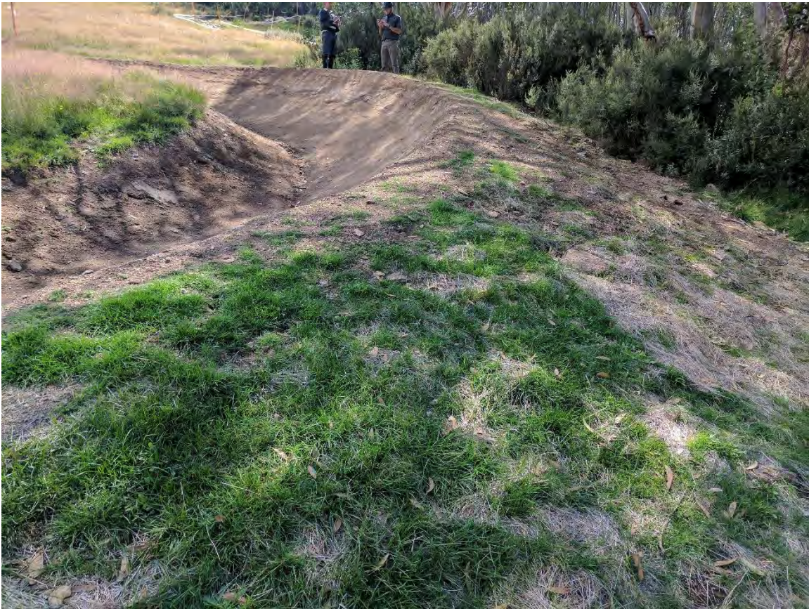
Figure 11: Section 6 - Relocation of the corner will allow for this berm to be located off the ski slope
